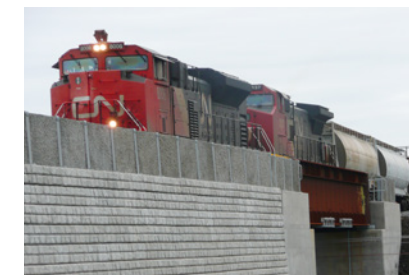
Handling Live Loads
